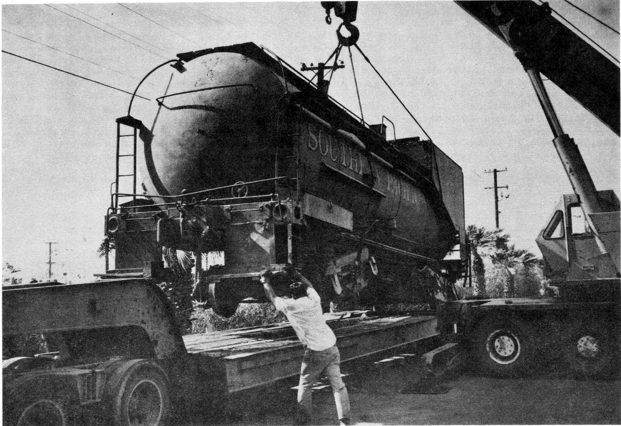
The tender was loaded, wheels and all, in a single lift at the fairgrounds using a hired 90 ton hydro boom shown here. The unloading at the museum was done with our own equipment but went just as smoothly. (Dale Prescott photo)
