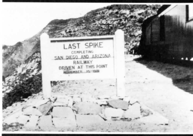
Site of the SD&A's Gold Spike ceremony in Carrizo Gorge (spelled "Carriso" by the railroad) about 1000 yards east of tunnel #8. Photo by S.D. Historical Society
